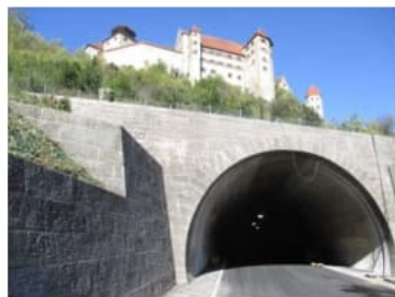
Portal Burgtunnel September 2015
